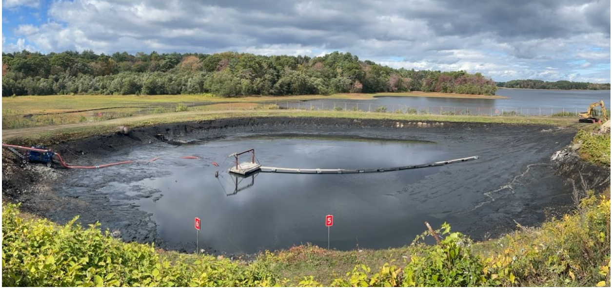
Residuals Lagoon at the Salem and Beverly Water Treatment Plant. Photo courtesy of Bradley Perron Deputy Director, Salem and Beverly Water Supply Board.
